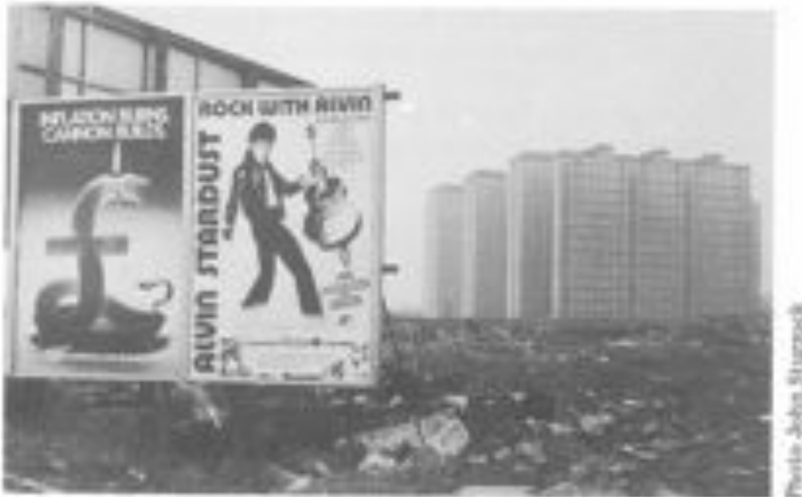
The Redroad flats, Glasgow, show that some council housing has fallen far short of its potential.
